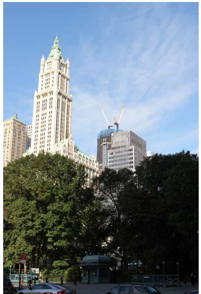
2011 - the construction of One World Trade Center Tower is under way Photos Bozena Pilat
