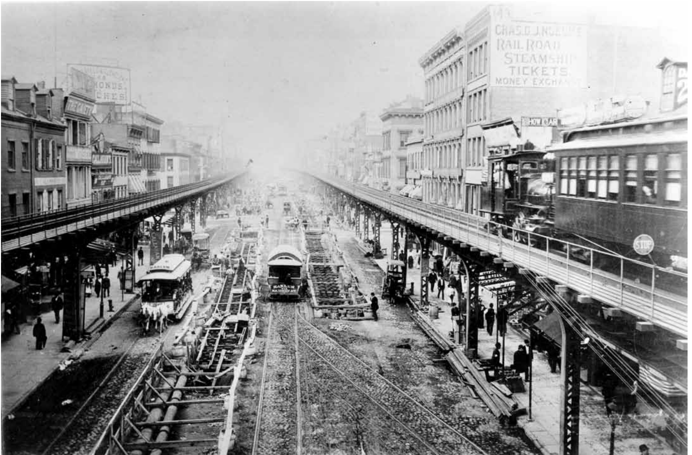
This photo showing a general view of the Third Avenue Line El train tracks, looking north up the Bowery from Grand Street, in New York City was taken in 1891 (5 years after the Modjeskis came to the United States.) On the west side of the street the cable car tracks are being installed.
