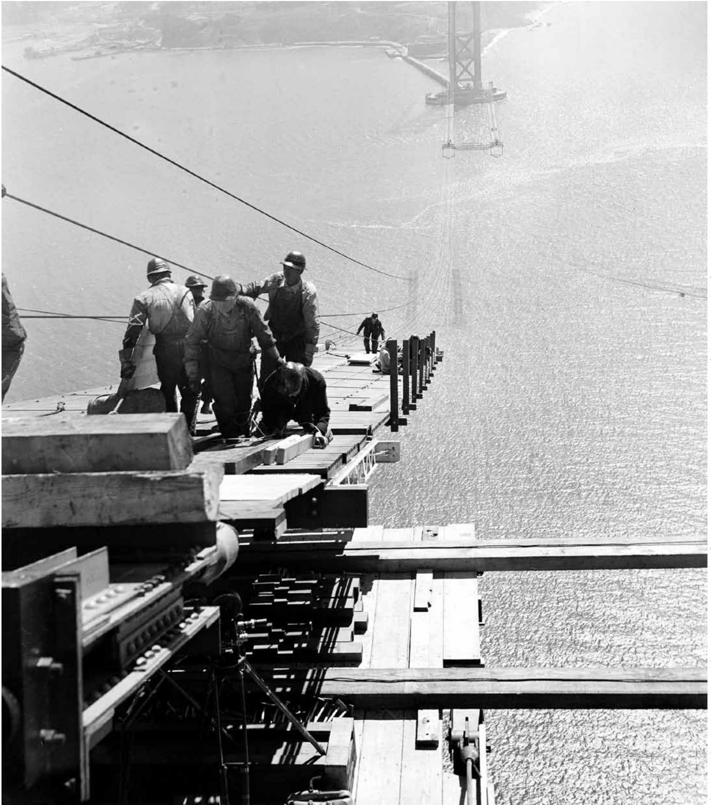
Workmen wearing steel helmets lay the catwalks for the Golden Gate Bridge in San Francisco, September 19, 1935. (AP Photo)
