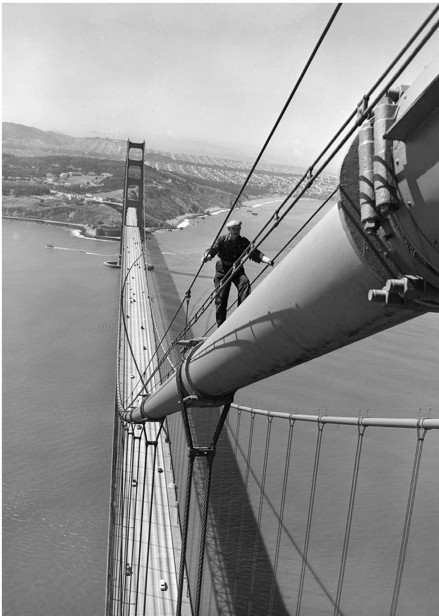
Bill Gaure, maintenance worker on the Golden Gate Bridge in San Francisco, nears the top of the north tower after nearly a half-mile uphill hike from the center of the span, May 15, 1952. In the background at center, is a residential area of San Francisco, and at upper left is part of the Presidio. The bridge was built right where the Pacific Ocean and San Francisco Bay meet. (AP Photo/Ernest K. Bennett)
