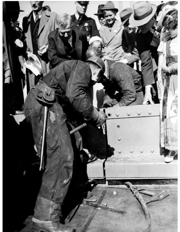
Ed Stanley drives the golden rivet to mark the completion of the $35,000,000 Golden Gate Bridge spanning the entrance to San Francisco Bay, April 29, 1937. Holding the rivet is Ed Murphy and leaning over them is Joseph B. Strauss, chief engineer of the project. (AP Photo)
